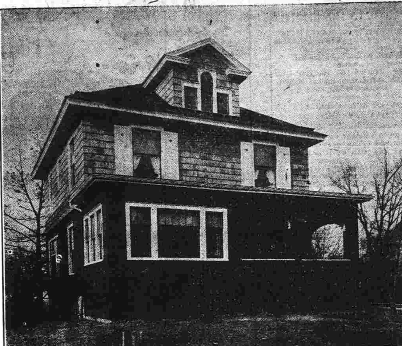
The sun parlor was the result of modernization. Note how the shingles have aided the appearance of the house.
